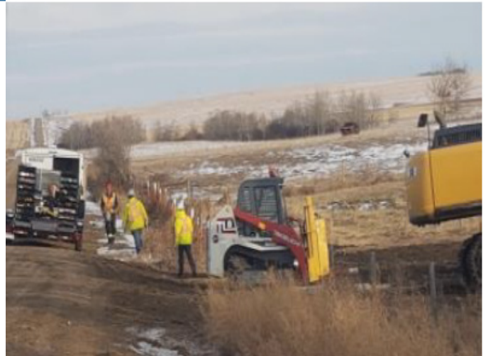
Fencing crew putting up posts and wire – SF 52 – Nov 14, 2018
