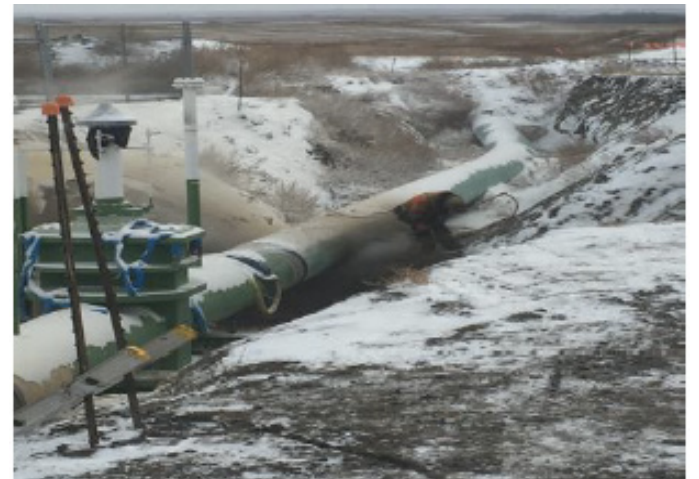
Hydro vac cleaning work area– SF 59 – Nov 16, 2018
