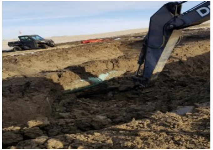
Excavator spooning under pipe – SF 22 - Nov 13, 2018
