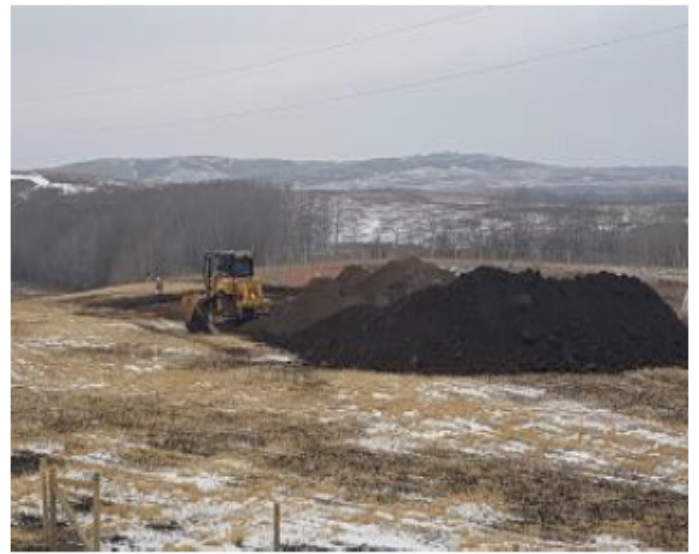
Ovality completed – SF 29 – Nov 15, 2018
