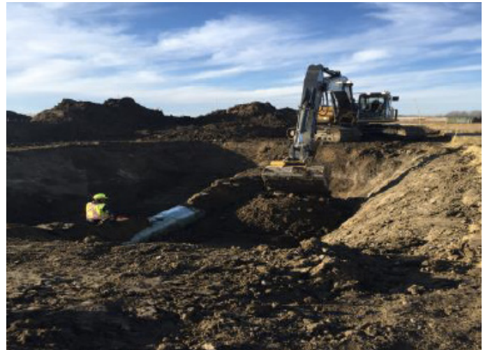
Ovality backfill – SF 24 – Nov 14, 2018
