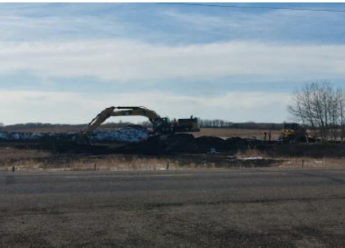
Transition topsoil replacement – SF 17 – Nov 14, 2018
