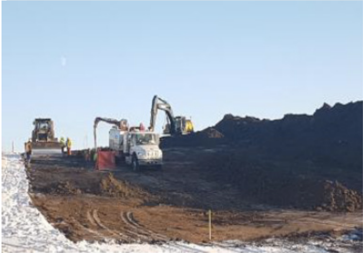
Hydro vac locating pipe – SF 30 – Nov 16, 2018
