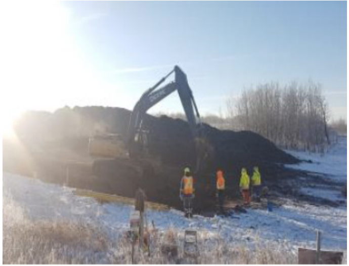
Excavator digging bell hole– SF 30– Nov 17, 2018
