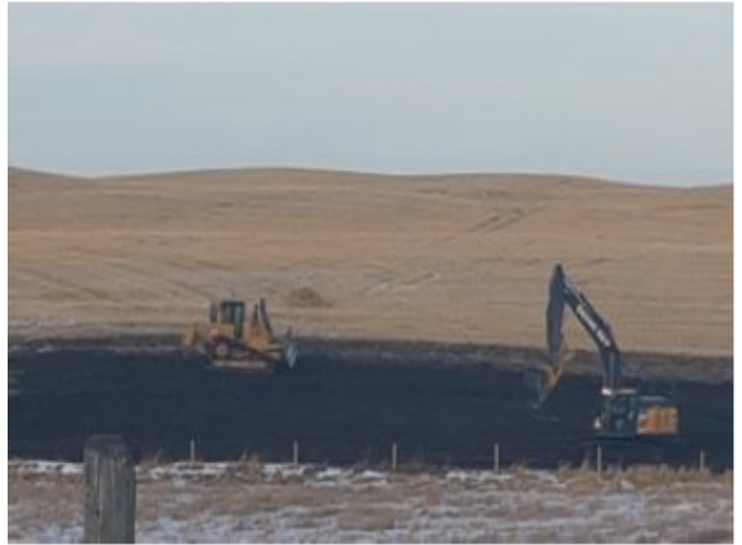
Dozer and excavator backfilling ovality dig– SF 75 – Nov 13, 2018
