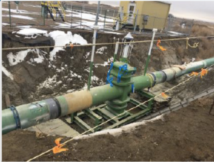
UT inspection site – SF 59 – Nov 15, 2018
