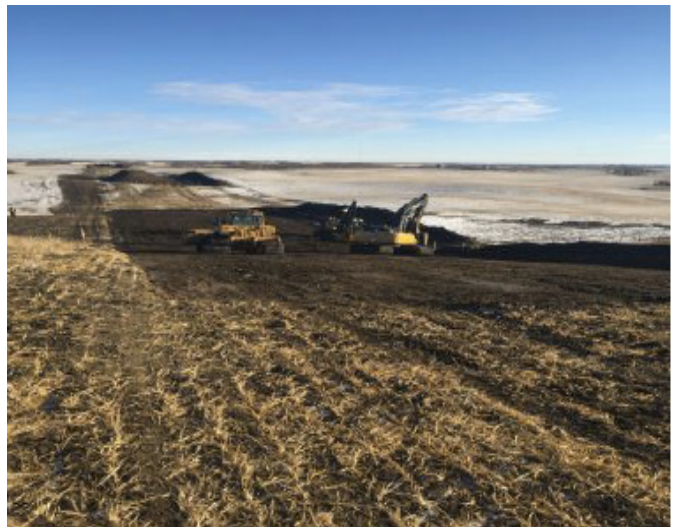
Replacing backfill– SF 22 – Nov 13, 2018
