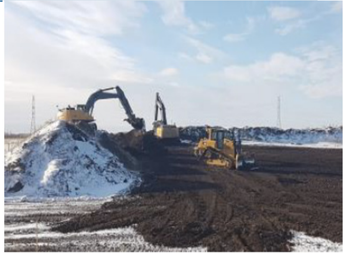
Excavator and dozer spreading top soil – SF 34 – Nov 16, 2018
