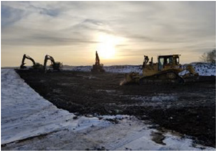
Excavator bailing ovality cuts to dozer - SF 25 – Nov 17, 2018
