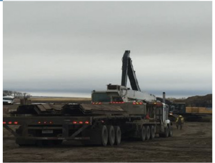
Valve tie-in sheet piling delivered – SF 61 – Nov 15, 2018
