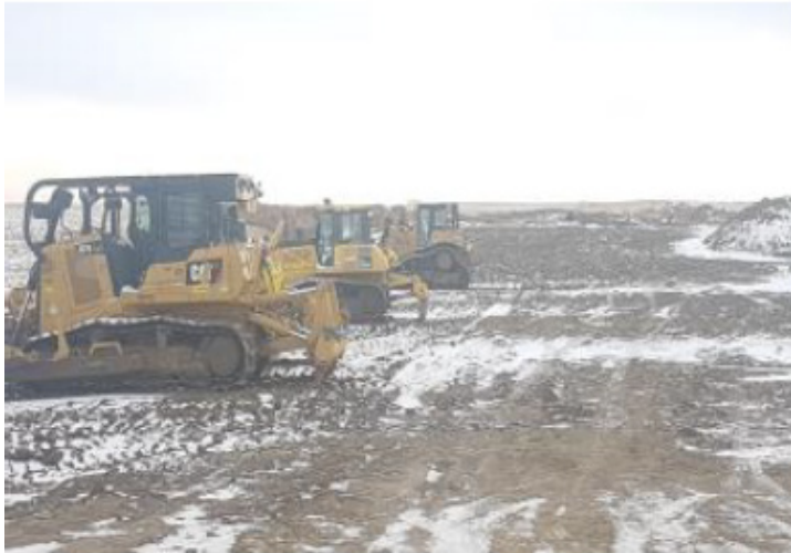
Equipment ready for removal – SF 44 – Nov 13, 2018
