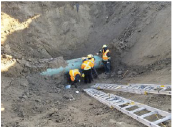
Laborers cleaning pipe – SF 27 - Nov 17, 2018
