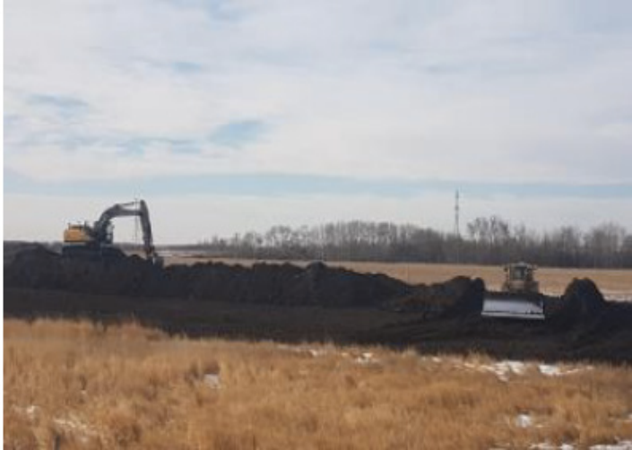
Excavator and dozer replacing topsoil – SF 34 – Nov 14, 2018
