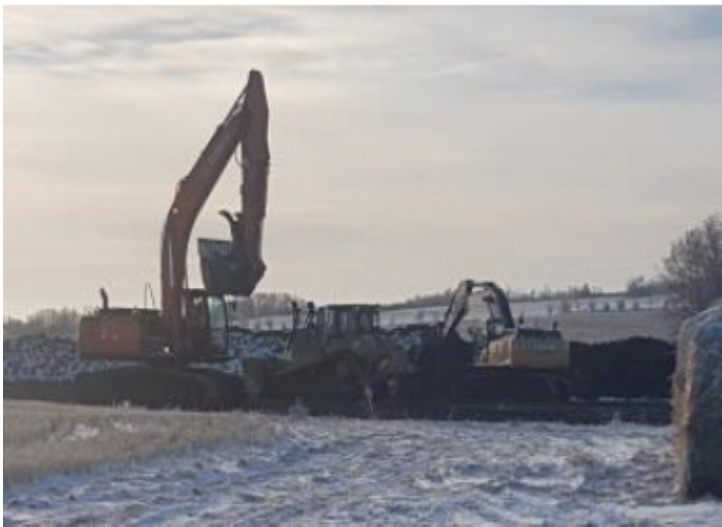
Dozer and excavator spreading and compacting– SF 25 – Nov 17, 2018
