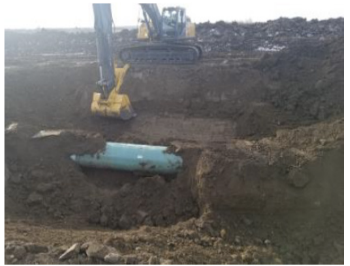
Excavator shading pipe – SF 23 – Nov 14, 2018
