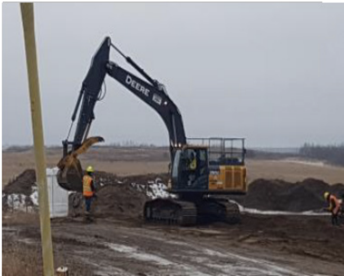
Excavator pulling topsoil back on ROW – SF 17 - Nov 15, 2018
