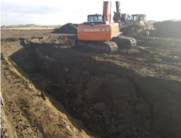
Excavator digging ditch for ovality – SF 25 – Nov 14, 2018
