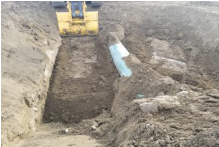
Excavator shading pipe – SF 22 – Nov 13, 2018
